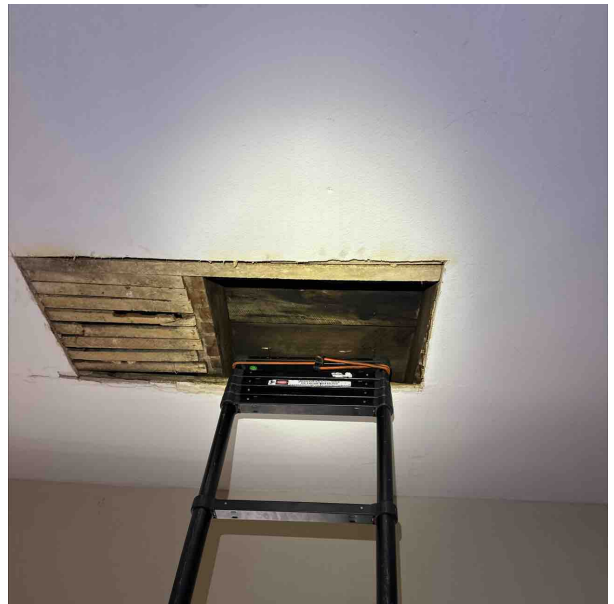
Caption: inside ceiling
